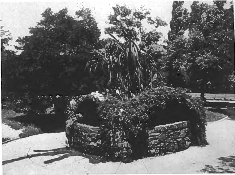
Figure I-31: Fresh-water fountain installed by the Park Commission to the west of the mansion, c. 1895. (Courtesy of Maryland Historical Society). cpI-31grotto
