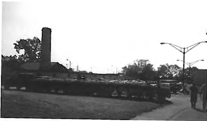
Figure II-32: Golf course and city maintenance buildings in conflict with parking and visitors. (LANDSCAPES LA•Planning•HP). cpII-31golfpkg
