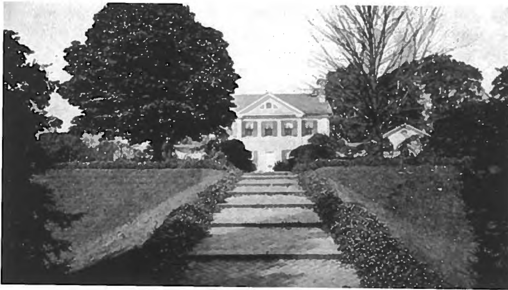
Figure I-23: Image showing brick walk leading up to the east side of the Mount Clare mansion from Washington Blvd. c. 1895. (Courtesy of Mount Clare Mansion Collection). cp1-22axissteps
