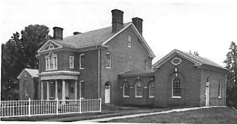
Figure II-24: West facade and forecourt of Mount Clare mansion. (Courtesy of SHPO, photo by Peter E. Kurtze). cpII-23mansw
