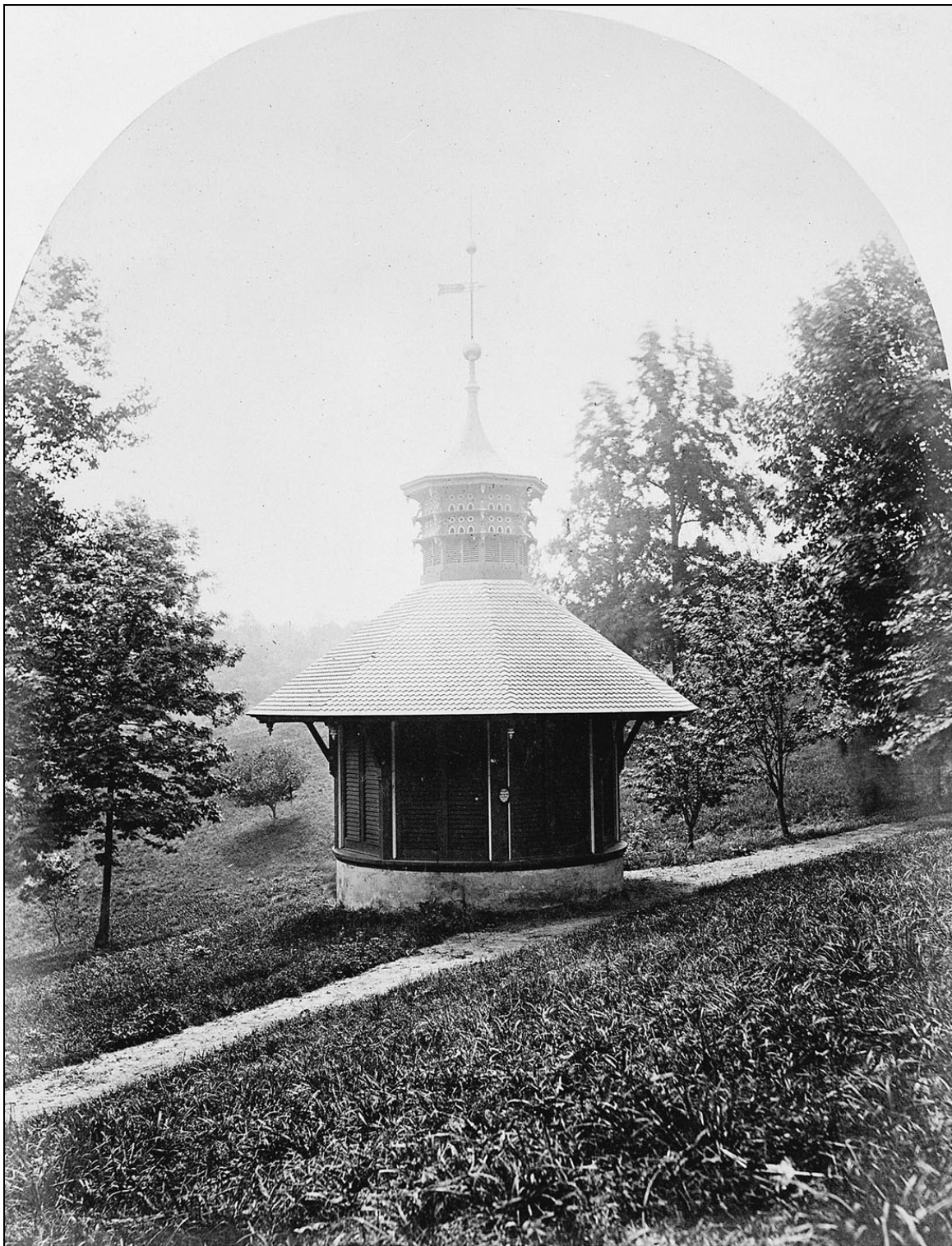
Figure II.2 Historic image on the Crimea grounds of an ornamental Gazebo with louvered doors, while small openings in the cupola appear to indicate a pigeonaire function, circa 1875 photograph. Courtesy Maryland Historical Society, Crimea-R-Gazebo-MHS-Z24-1178.
