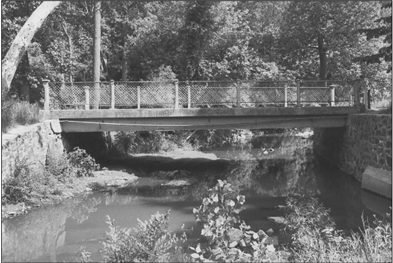
Figure II.8 A reconstructed bridge over Dead Run using the Winans era railings. Courtesy National Register Nomination, Kurtze, CRI-R-Bridge.
