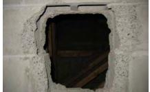
Figs. 12, left; and 13, right. Views in the roof truss area. Left: unprotected access hole through fire wall on west side. Right: unprotected access hole through fire wall on east side.
