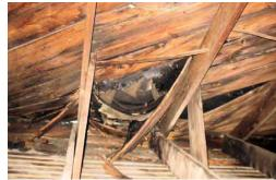
Figs. 18 left; and 19, right. Views in the roof truss area, East Wing. Left: termite damage at north side; extent extends approximately five bays. Right: water damage to sheathing, and missing sheathing, south side.
