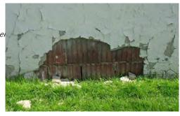
Figs. 9, left; and 10, right: Left: Detail at wall and roof of East wing, south side, showing plaster condition and damage to roof sheathing near gutter (missing). Right: West wing, north elevation, showing an area where the stucco is delaminating and actually missing from the back-up clay tile wall system.
