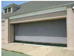
Figs. 3, left; and 4, right. Left: EIFS surface on North elevation of the central portion of the Pool house. Ball practice is causing damage on the surface of the stucco. Right: Central wing, south elevation; the manual-operated coil down door is currently unable to fully close.
