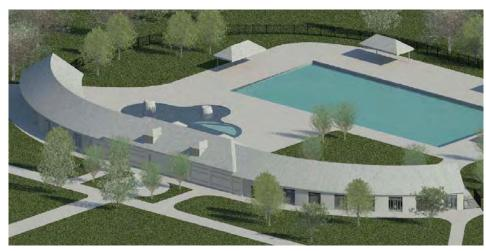
Image 9 – Northwest bird's-eye view of Option 2. Walls at existing window locations have been removed and openings are gated at park side.
