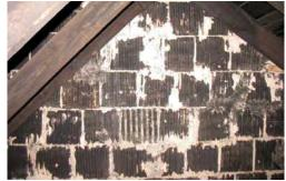
Figs. 16 left; and 17, right. Views in the roof truss area, West Wing. Left: damaged and missing sheathing, north side of west wing, near end wall. Right: clay tile gable end wall.
