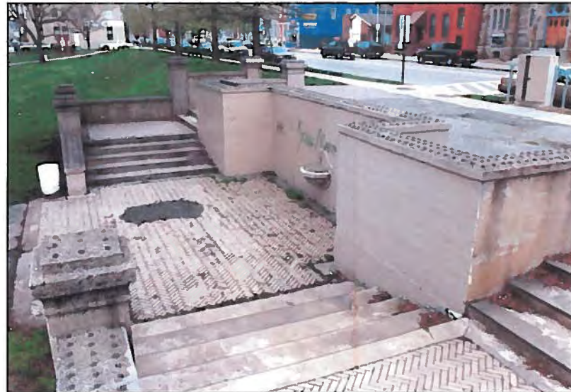
Image 5: Center grand staircase on Fort Avenue. Note herringbone pattern of brick and fountain on lower retaining wall.
